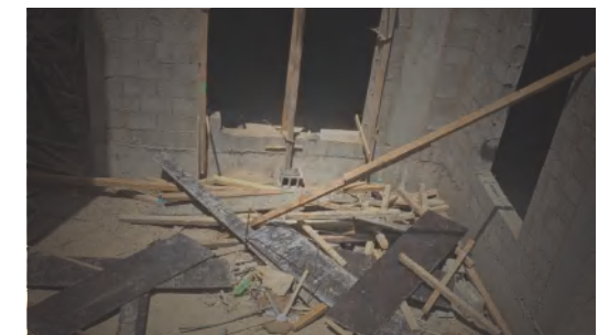
Timber Formwork on Site
