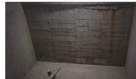
Timber Formwork Forming Effect
